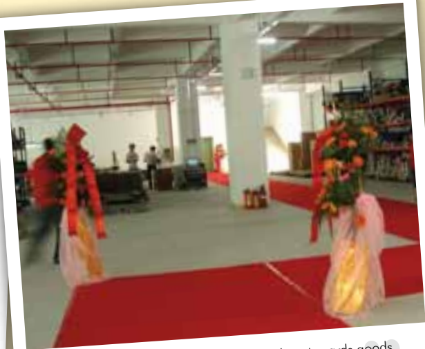
Ground floor – bulk materials store looking towards goods in-out area and goods lift
